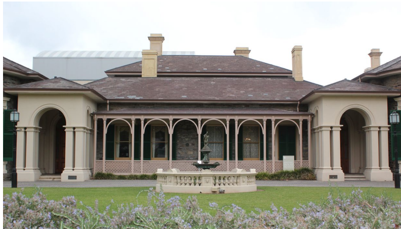
Front view of Ayers House, 2011 Courtesy of History Trust of South Australia
